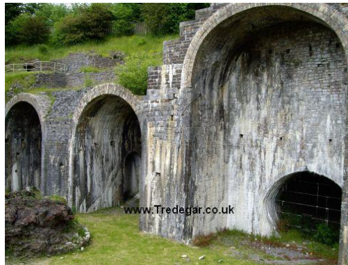
Part of the original furnace in Tredegar
